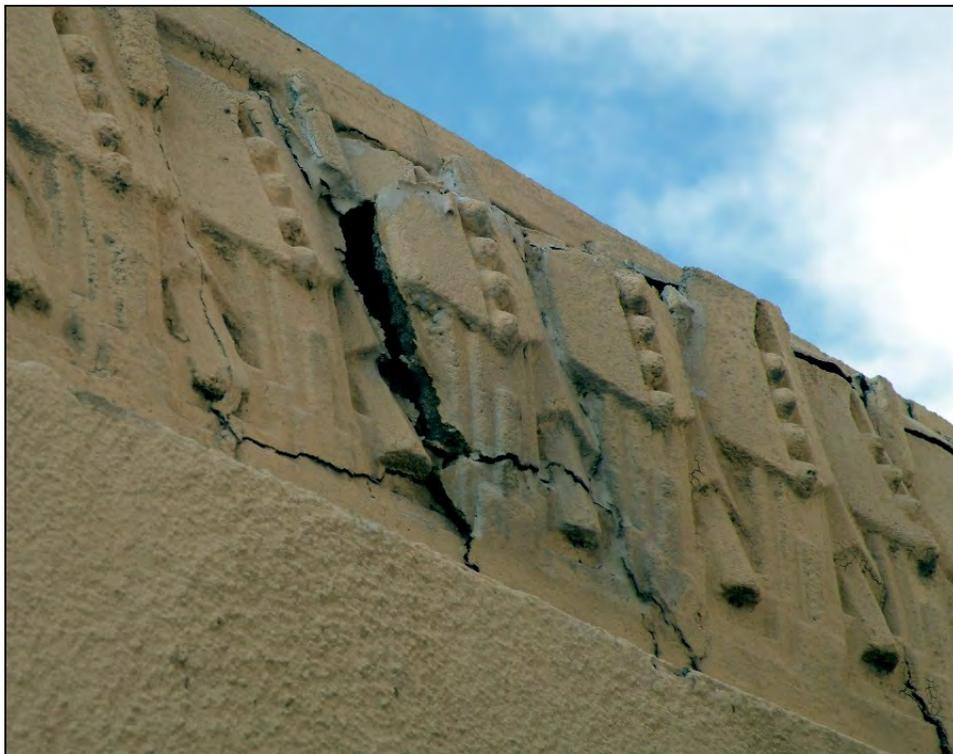
**Figure 18:** Typical decorative cast stone damage.
