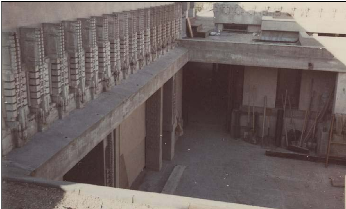
Figure 6: 1969 photograph of Porch removal. A new steel superstructure replaced the original porch in 1970. Photo Courtesy Hollyhock House archives.
