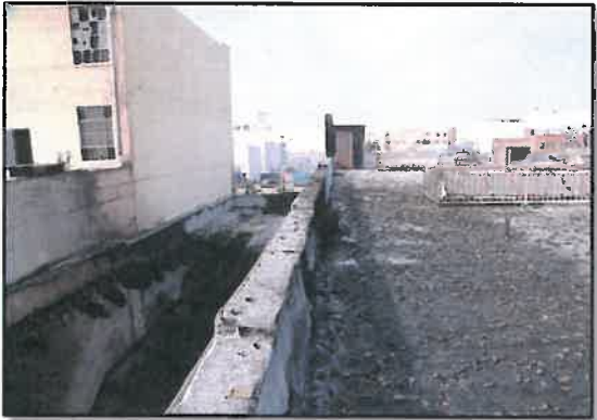
Perspective looking at Bravo rooftop
