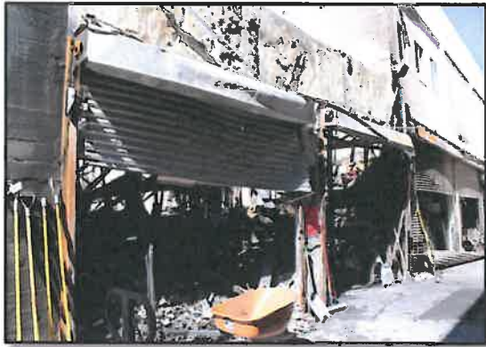
Charlie side looking towards the Bravo exposure
