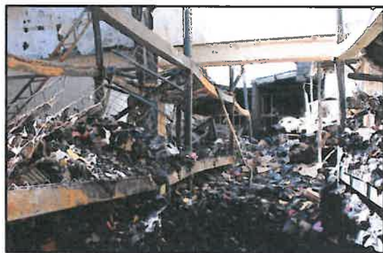
Charlie side looking into Unit A
