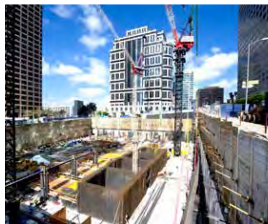
PHOTO ABOVE: The Intercontinental Wilshire/Grand under construction
