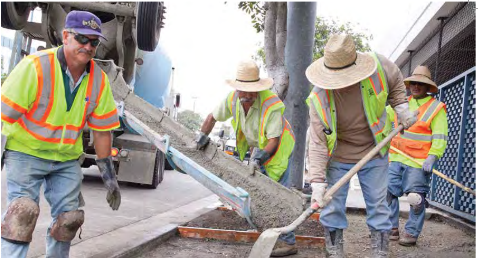
PHOTO ABOVE: Los Angeles Department of General Services replacing damaged sidewalks around the LACC in June 2014
