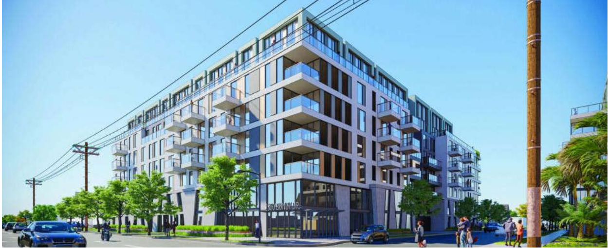
View of 2301 Bundy looking southwest
