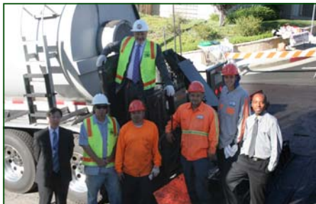
Councilman Zine with the Bureau of Street Services staff including Chi Ming Gong, James Duncan, and the slurry seal crew
