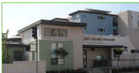
The completed Hart Village project in Canoga Park
