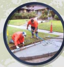
CURB & GUTTER REPAIR
