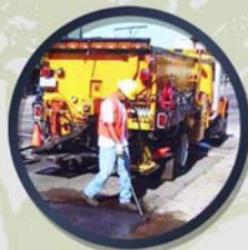
SMALL ASPHALT REPAIR
