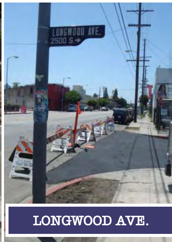
Longwood Ave. gets slurry sealed
