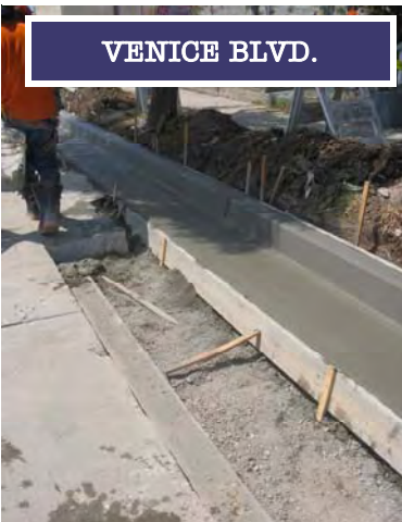
Sidewalk repair along Venice Blvd.
