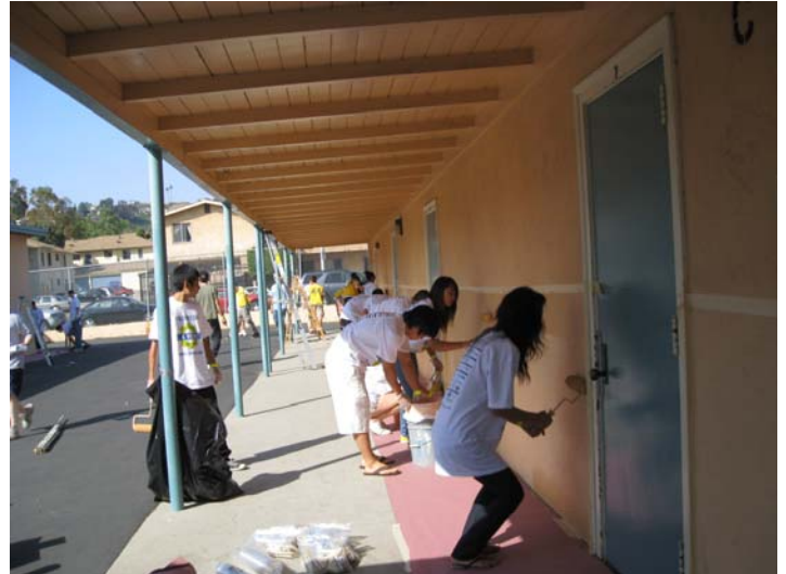
LA Works volunteers repainting Hillcrest Drive Elementary School
